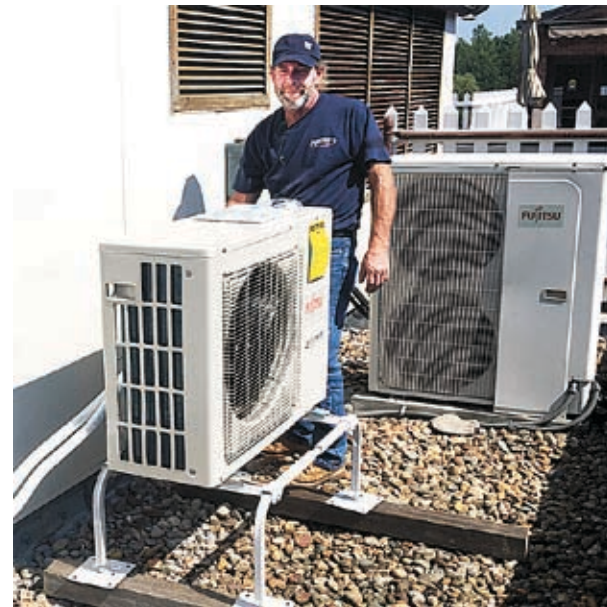
Paradigm HVAC technician William McGrath installs the new outdoor units.
