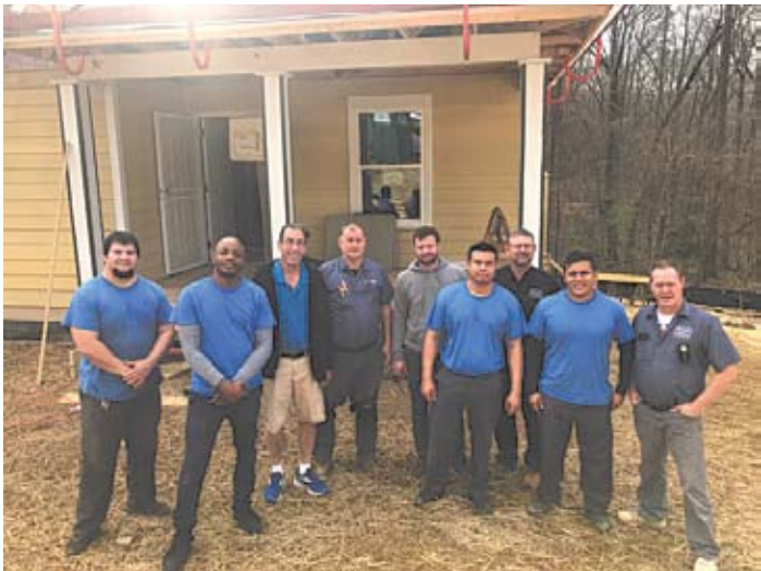
Central Heating and Air build team.
